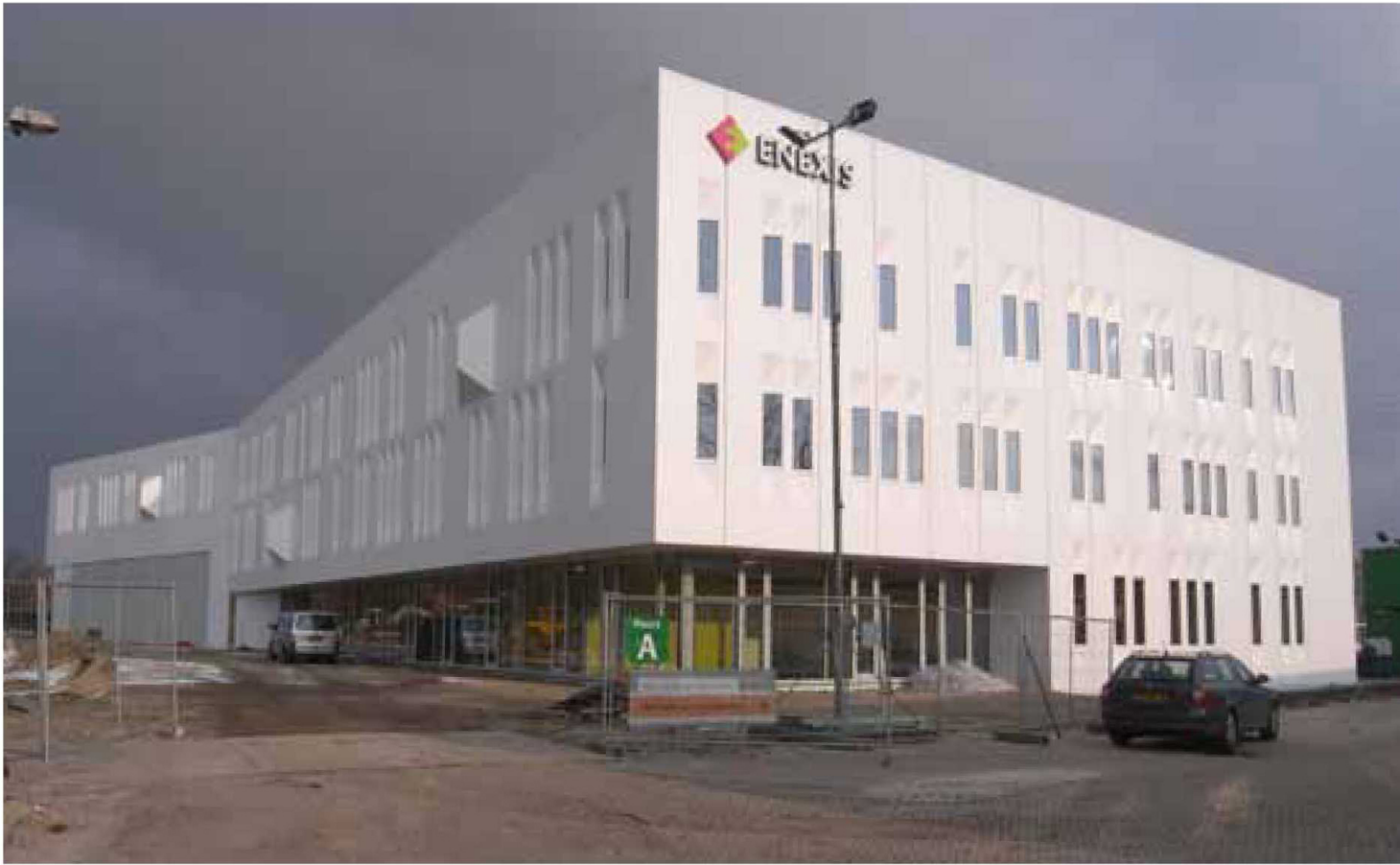
Regional office Enexis in Zwolle under construction
