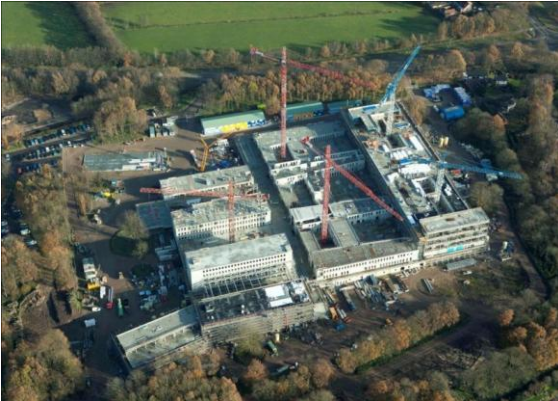
MEANDER HOSPITAL UNDER CONSTRUCTION
