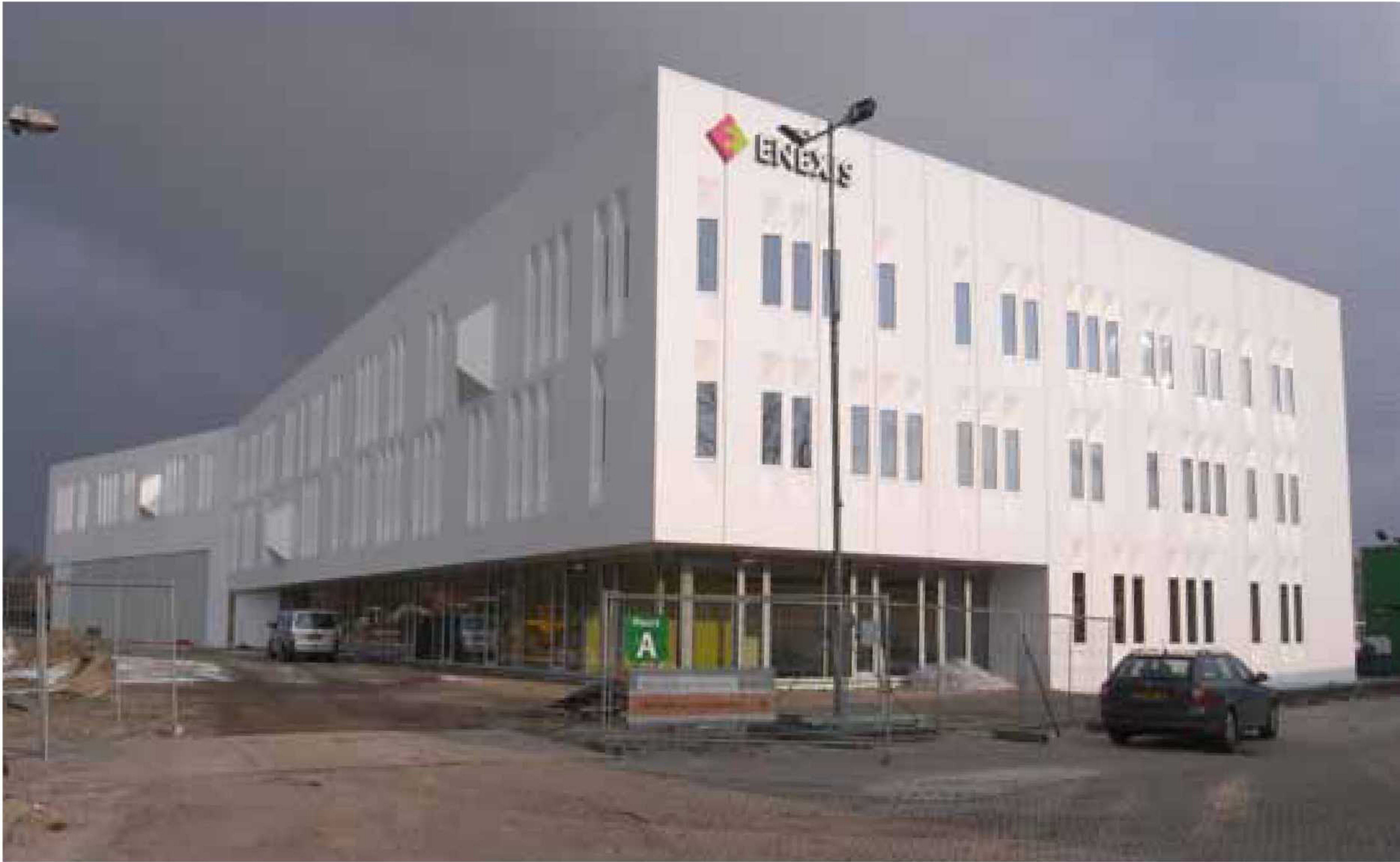
Regional office Enexis in Zwolle under construction
