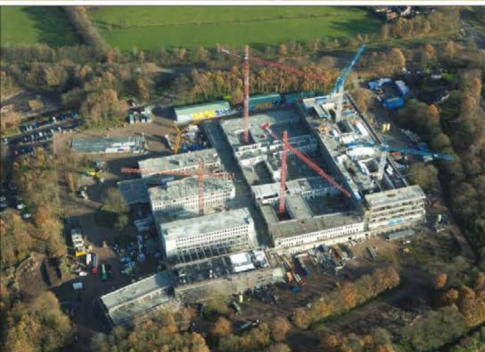
MEANDER HOSPITAL UNDER CONSTRUCTION
